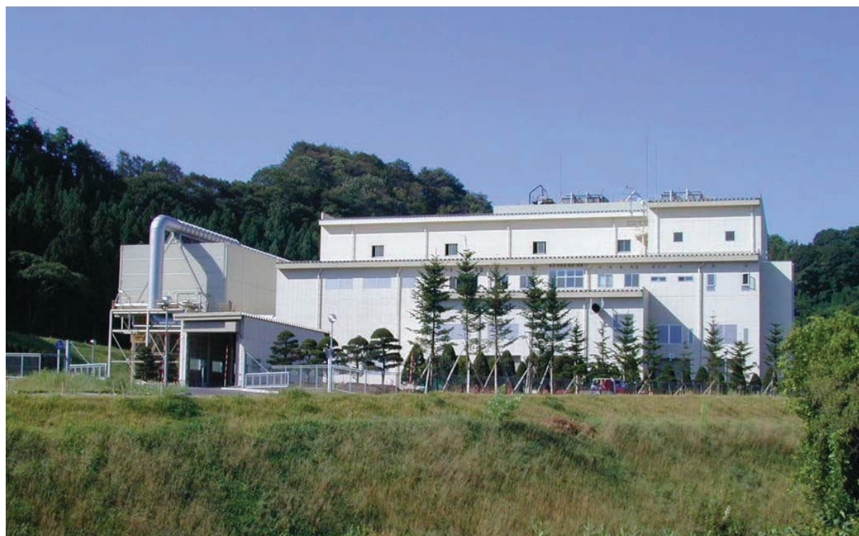
Figure 82. TwinRec facility in Aomori, Japan
